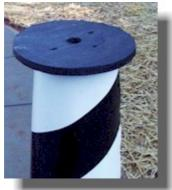
**Step 6.** Fasten 10" round plywood top on center of top wood donut as shown in picture on left. Use 4 wood screws through the plywood into the wood below.
